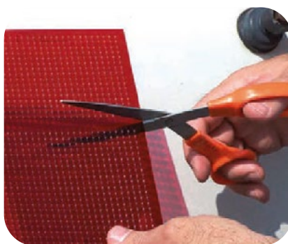
2. Cut the repair panel
